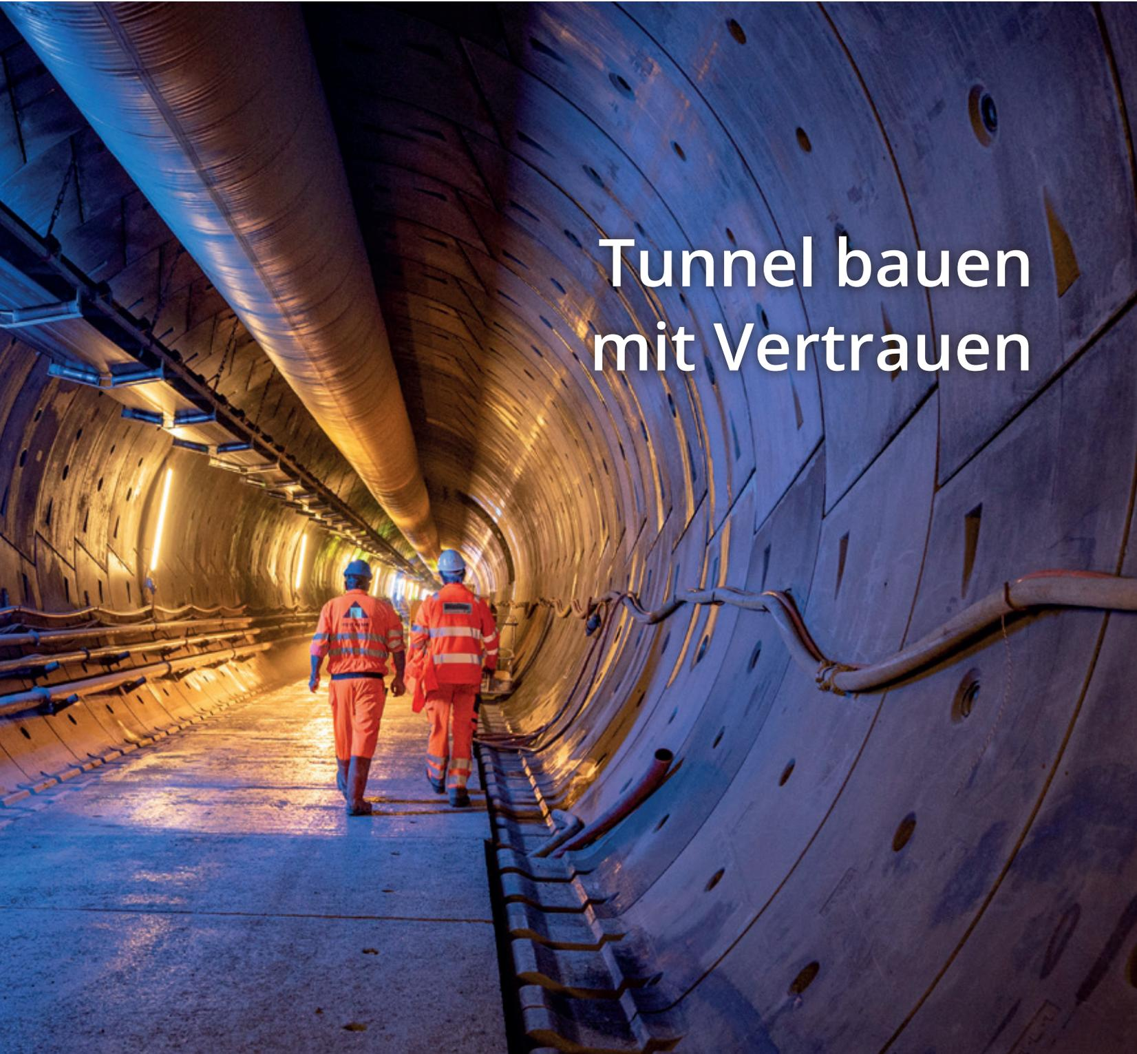
A photograph of a tunnel under construction. Two workers in orange safety suits and blue hard hats are walking away from the camera down the center of the tunnel. The tunnel walls are lined with large, curved metal segments, and a large, flexible pipe runs along the top. The floor is concrete, and the lighting is warm and focused on the workers.
